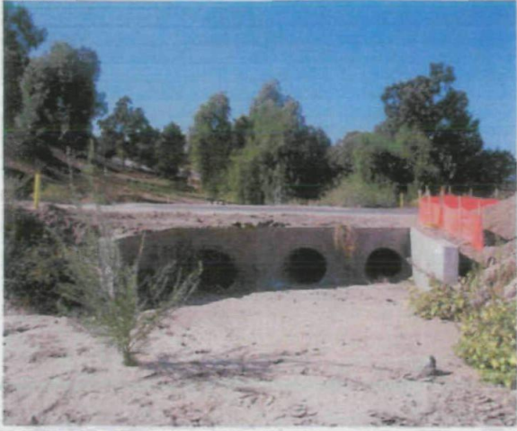
Figure 1. Looking downstream towards the culvert and Santiago Road.
