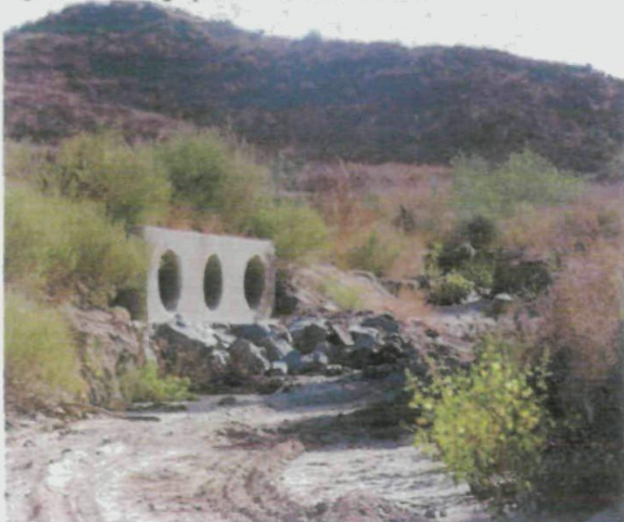
Figure 5. Looking upstream at culvert outlet.
