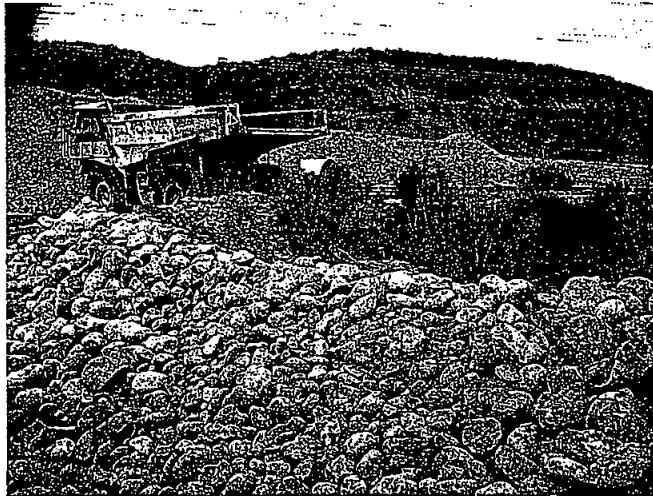
11. A rock berm that overlooks Carroll Canyon Creek on the east side of the facility.
