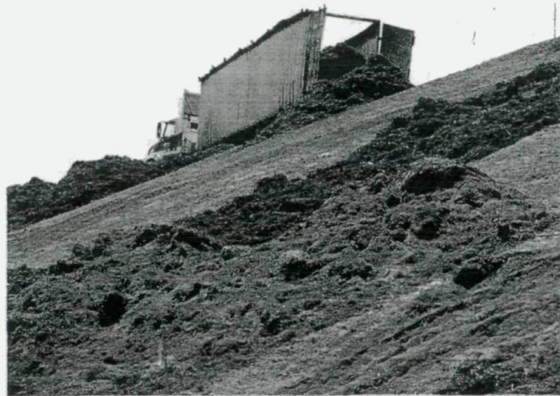
Contaminated green waste being received during inspection.
