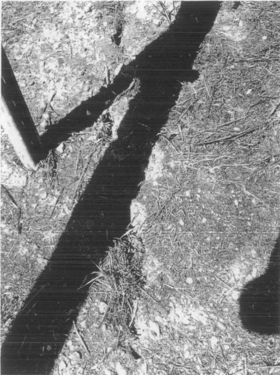
Crack in landfill CAP (see location on aerial photo)
