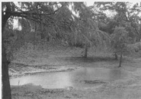
Photograph 2 – ASL cover ponding
