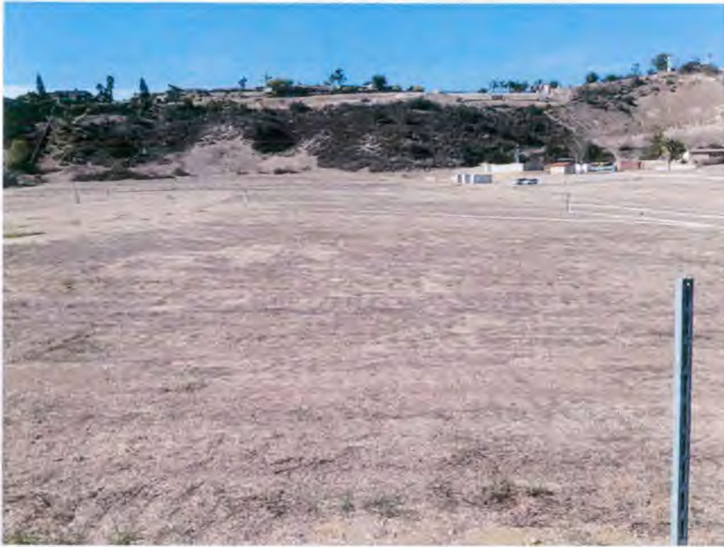
Figure 7- Landfill Cover Facing West
