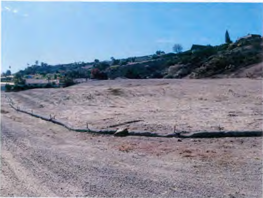
Figure 1- Soil Stockpile with surrounding BMPs
