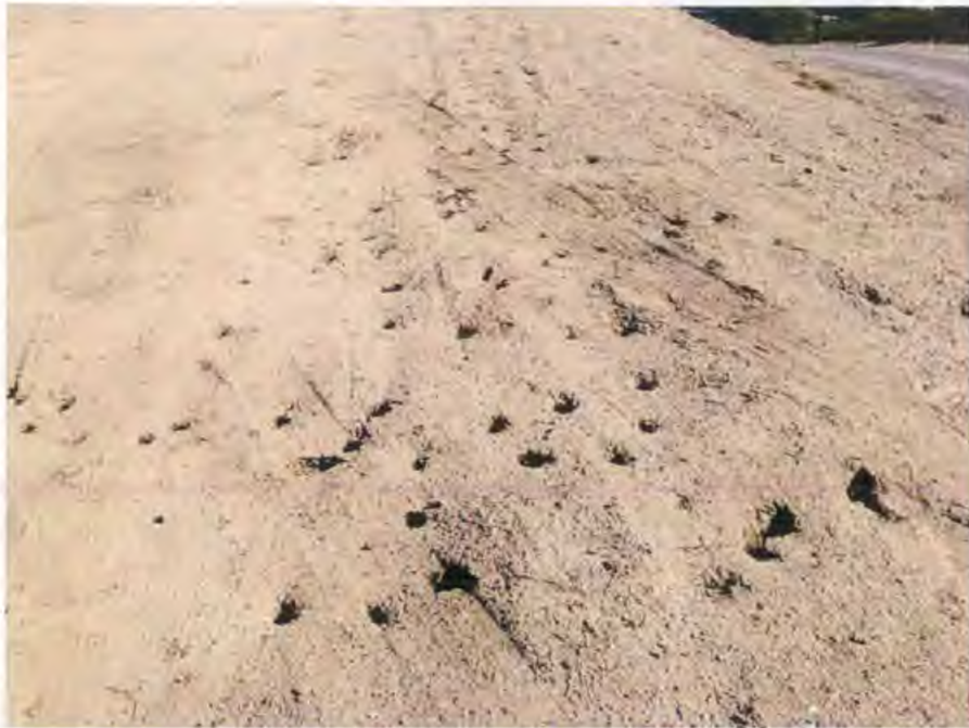
Figure 5- Southeast Landfill Slope
