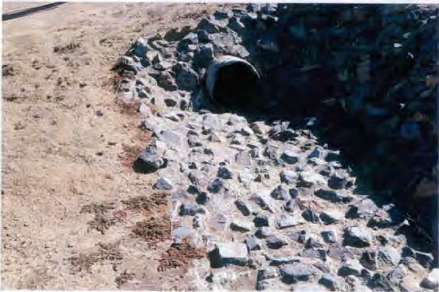
Figure 2- Southern Perimeter Drain
