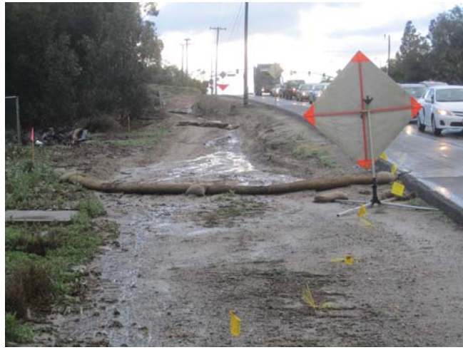
Time: 1030 By: D. Carlin View of area behind ECR curb line just south of Chestnut. BMP's intact, prior to being supplemented. No runoff identified from this area.
