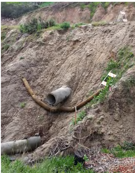
Photo 11 Lack of perimeter controls, inadequate run-on controls, lack of erosion in conjunction with sedimentation controls. (view is south of Photo 10 in the unnamed tributary to Agua Hedionda Creek and Agua Hedionda Lagoon).
