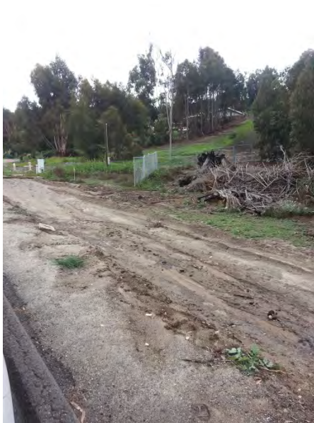
Photo 13 Lack of perimeter controls, lack of run-on controls, lack of erosion controls, lack of erosion controls in conjunction with sedimentation controls, and lack of soil stabilization controls. (view at south end of the site located on the west side of El Camino Real looking south toward inlet structure shown in Photo 16). This photo documents rilling evidence of erosion on this portion of the site due to an overall lack of perimeter controls, erosion and sedimentation controls.
