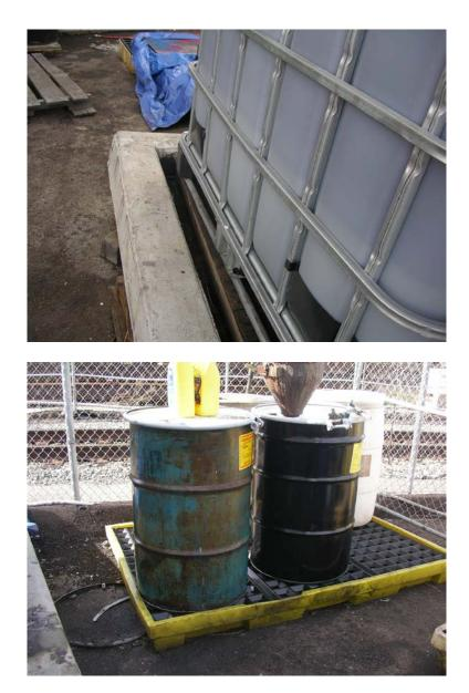
Photo 10. Secondary containment of bilge water cubes with water.
