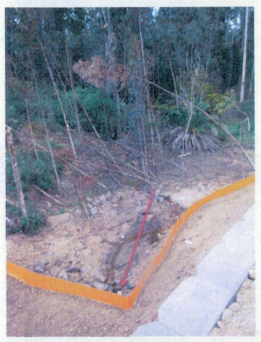
Photo 3 - Unnamed tributary entering pipe inlet. Direction of flow in red.
