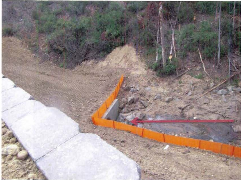
Photo 1 – Pipe inlet from above. Direction of flow in red.
