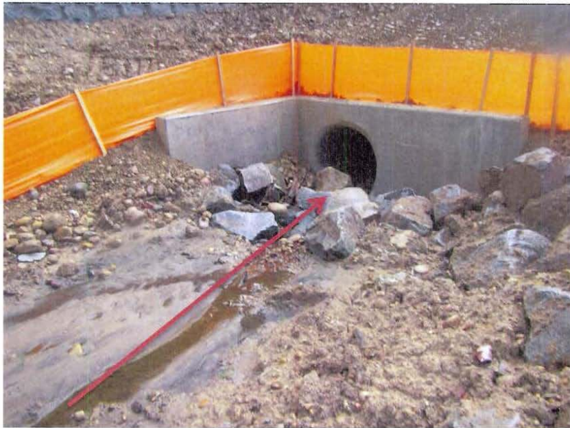
Photo 2 – Pipe inlet looking northwest. Direction of flow in red.
