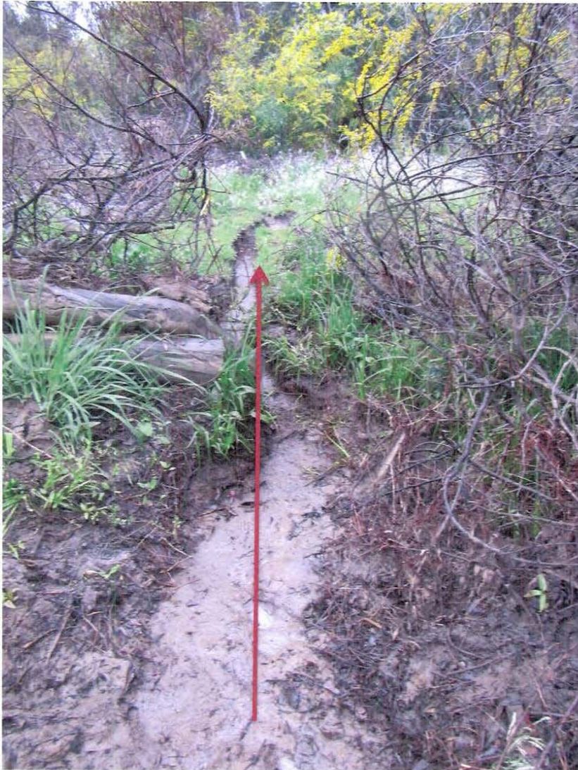
Photo 6 – Area in which pipe outfall flows north into tributary. Direction of flow in red.
