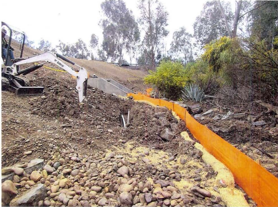
Photo 4 – Pipe outlet, photo facing northwest.
