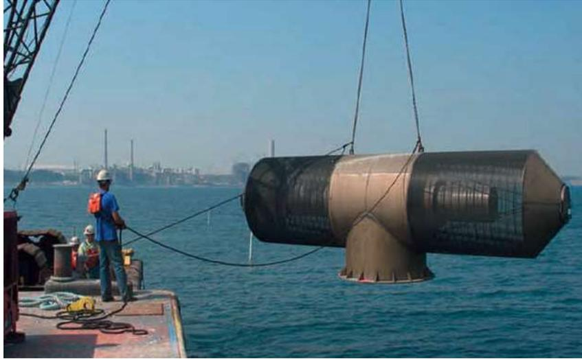
**Figure 8. Passive wedgewire screen being installed (image courtesy Aqseptence)**
