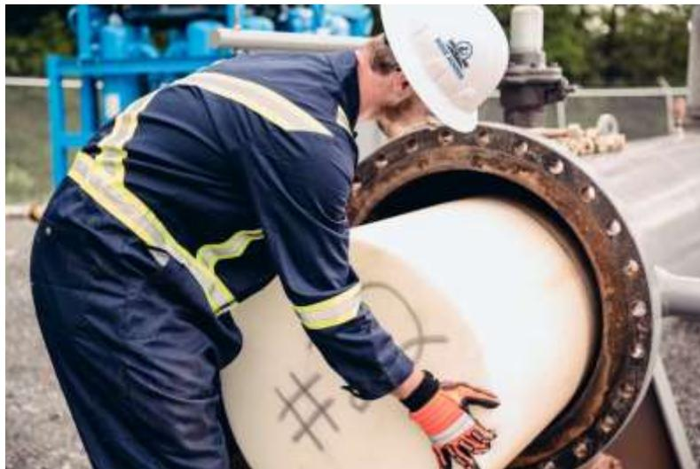
**Figure 5. Pig insertion for physical pipe cleaning (image courtesy Ridge Runner Pipeline Services).**
