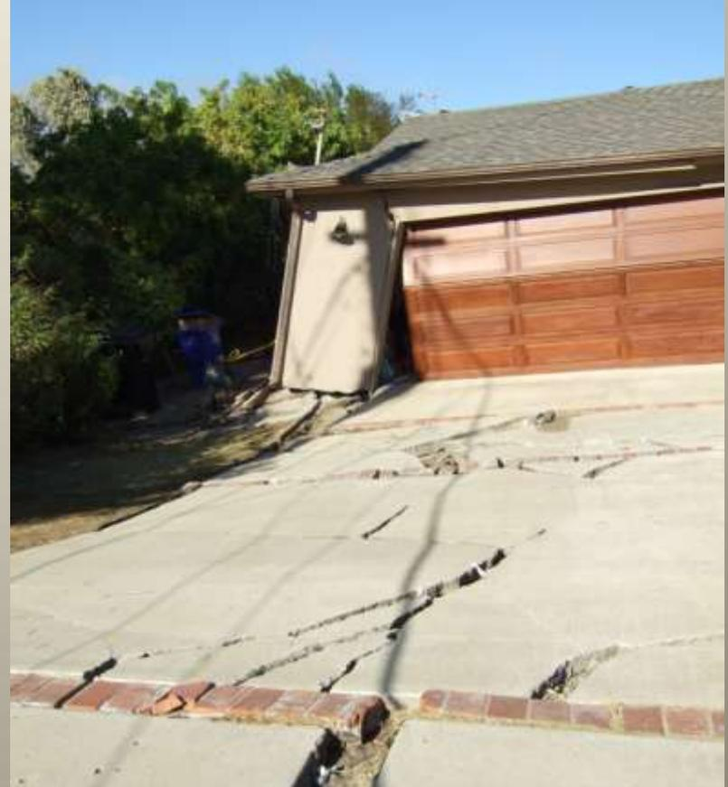
Water in Clay Soils-Ardath Shale-Clay Soil Group D
