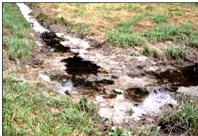
FIGURE 3-32 Failing sanitary sewer, causing upwelling of sewage through soil, and draining to gutter and then to storm drainage system. SOURCE: Robert Pitt, University of Alabama.
