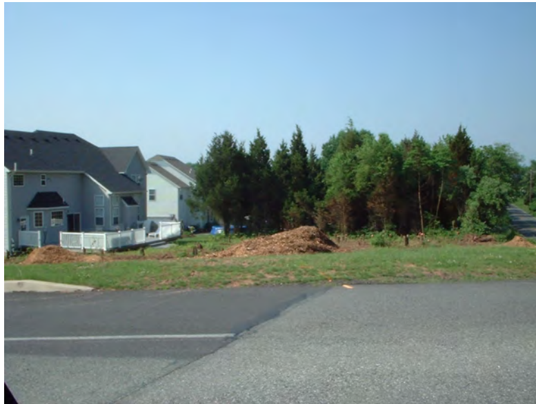
FIGURE 5-52 Wooded conservation area stripped of trees. Note pile of sawdust. SOURCE: Robert Traver, Villanova University.
