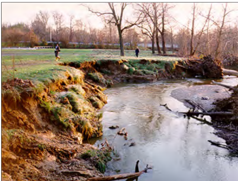
FIGURE 1-5B A destabilized stream in Vermont. SOURCE: Courtesy of Pete LaFlamme, Vermont Department of Environmental Conservation.
