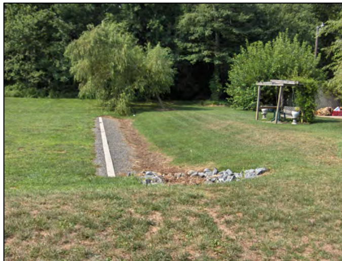
FIGURE 5-11 Level spreader. SOURCE: Robert Traver, Villanova University.
