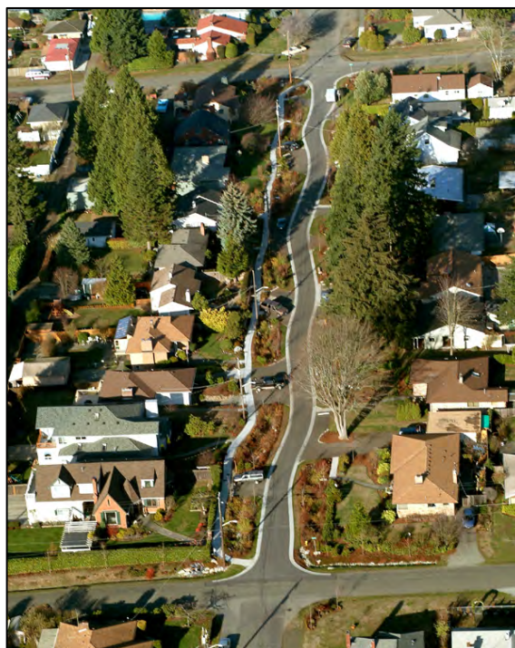
FIGURE 5-6 110 th Street, Seattle, part of the Natural Drainage Systems Project. This location exhibits several elements of impervious cover reduction. In particular, vegetated swales were installed and curbs and gutters removed. There are sidewalks on only one side of the street, and they are separated from the road by the swales. The residences' rooftops have been disconnected from the storm-drain systems and are redirected into the swales. SOURCE: Seattle Public Utilities.
