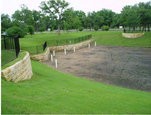
FIGURE 5-45 Austin sand filter. SOURCE: Robert Traver, Villanova University.
