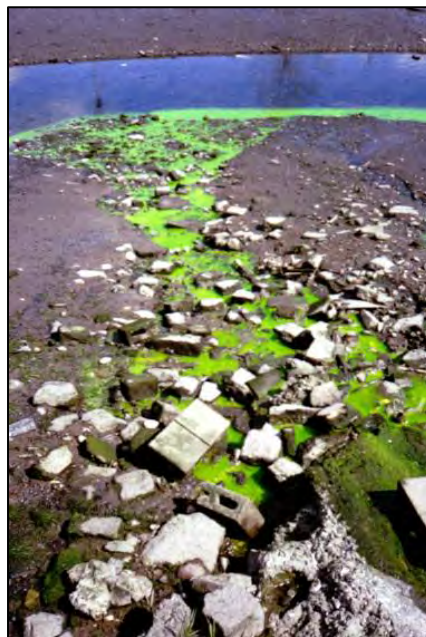
FIGURE 3-33 Dye tests to confirm improper sanitary sewage connection to storm drainage system. SOURCE: Robert Pitt, University of Alabama.
