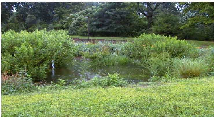
FIGURE 5-19 Retrofit bioinfiltration at Villanova University immediately following a storm event. SOURCE: Robert Traver, Villanova University.
