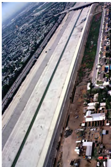
FIGURE 3-25 Example of a channelized urban stream for maximized flood conveyance and geomorphic stability (Los Angeles River, California). SOURCE: Robert Pitt, University of Alabama.
