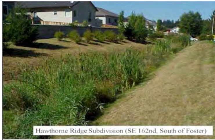
FIGURE 5-16 Vegetated swale. SOURCE: PaDEP (2006).
