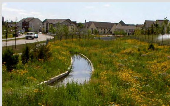
FIGURE 5-57 View of a sediment trap and porous landscape detention area in the central parkway spine of Heritage Park. The sediment trap in the center left of the photo was designed for ease of maintenance access by city crews with standard city maintenance equipment. SOURCE: Courtesy of the SRF Consulting Group, Inc.
