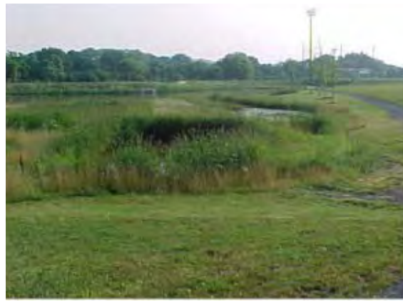
FIGURE 5-40 Constructed wetland. SOURCE: PaDEP (2006).
