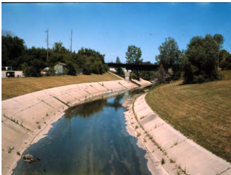
FIGURE 5-2 Concrete channel in Lincoln Creek, Milwaukee, Wisconsin. SOURCE: Roger Bannerman, Wisconsin Department of Natural Resources.
