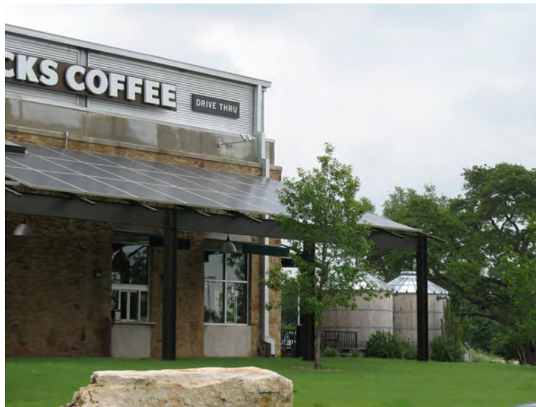
FIGURE 5-14 Rainwater harvesting tanks at a Starbucks in Austin, Texas. SOURCE: Laura Ehlers, National Research Council.
