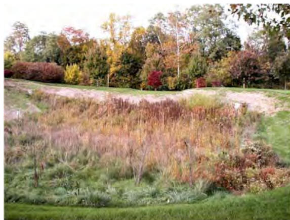
FIGURE 5-43 Dry extended detention pond. SOURCE: PaDEP (2006).
