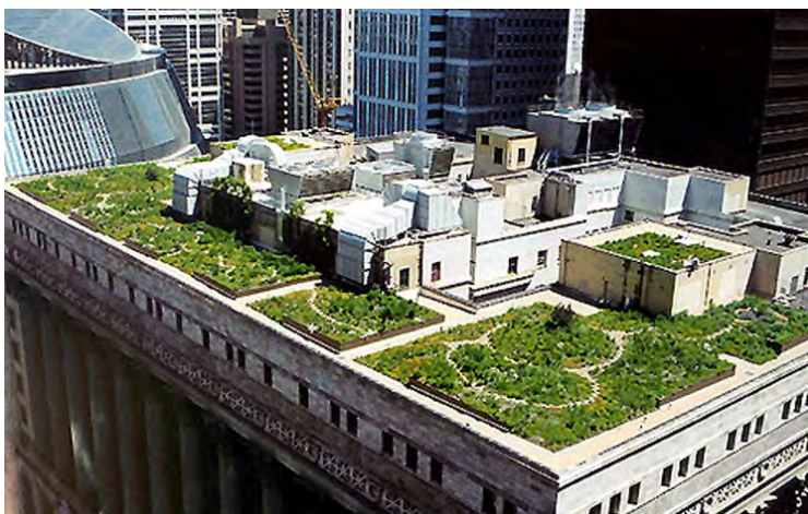
FIGURE 5-18 City Hall in the center of Chicago's downtown was retrofitted with a green roof to reduce the heat island effect, remove airborne pollutants, and attenuate stormwater flows as a demonstration of innovative stormwater management in an ultra-urban setting. SOURCE: Courtesy of the Conservation Design Forum.
