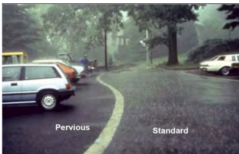
FIGURE 5-29 Porous asphalt. SOURCE: PaDEP (2006).
