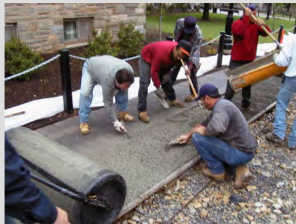
FIGURE 5-34 Infiltration bed under construction. Pervious concrete has functionality and workability similar to that of regular concrete. However, the pervious concrete mix lacks the sand and other fine particles found in regular concrete. This creates a significant amount of void space which allows water to flow relatively unobstructed through the concrete. This site was the first attempt at creating a pervious concrete SCM in the area, and there were construction and material problems. Since that time the industry has matured, and a second site on campus constructed in 2007 has not had any significant difficulties. SOURCE: Reprinted, with permission, from VUSP. Copyright by VUSP.
