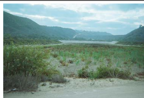
Existing sediment basins intercept runoff from Goat Canyon (background)
