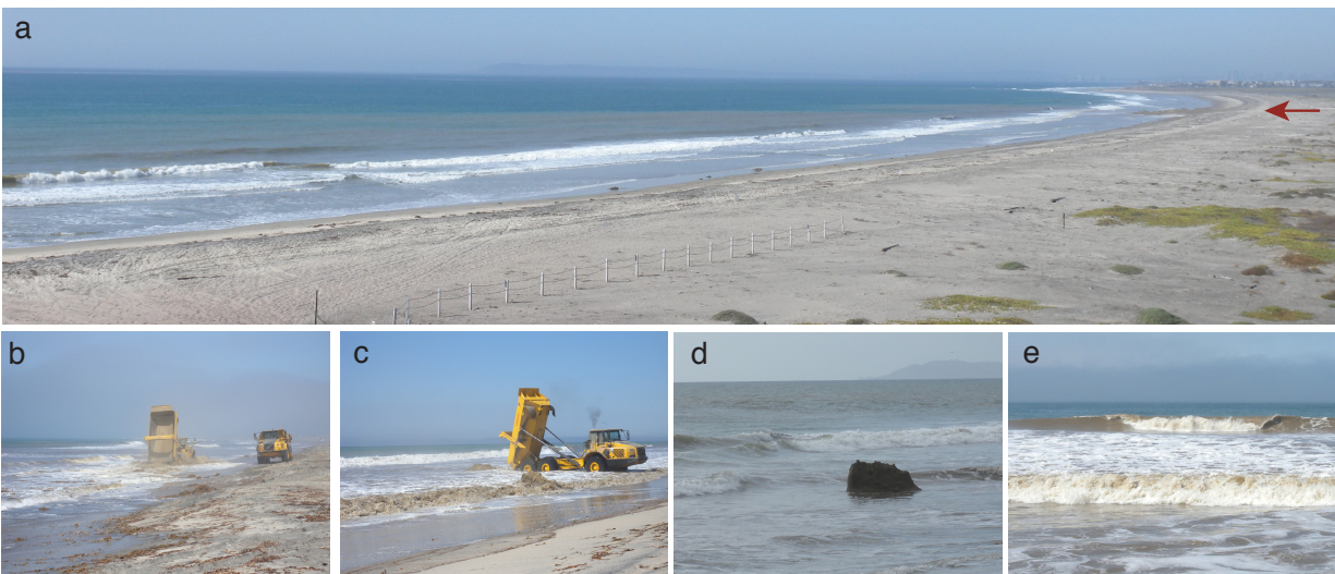
Figure 2. Photographs of the study site and sediment-nourishment project. (a) Overview perspective from the United States-Mexico border showing the sediment placement site (arrow) and southern-directed turbid plume on October 1, 2009, 1447 PDT. (b and c) Sediment placement within the swash zone. (d) A recently placed pile of sediment in the swash. (e) Turbid surf zone immediately adjacent to the sediment placement site.
