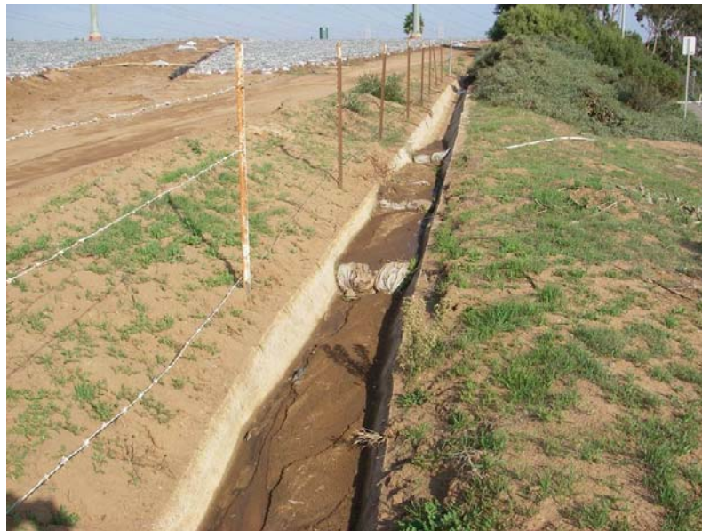
Figure R-5. Use of Sandbags near Strawberry Fields, Cannon Rd. near Interstate 5, Carlsbad Watershed.
