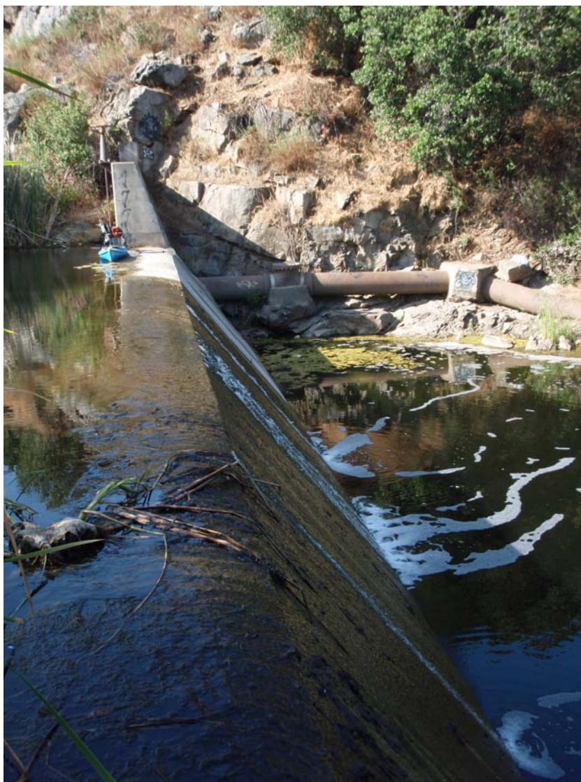
Figure 2-3. Los Peñasquitos Creek Surface Water Impoundment East of I-15
