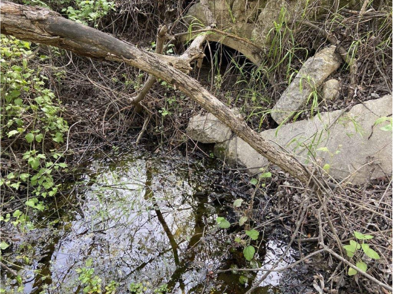
Outlet of pipe downstream from Pond 22/Permanente Creek
