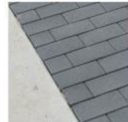
pavers with poured concrete
