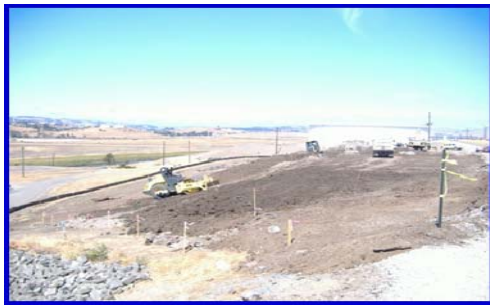
Photo #1 – Unit Closure Preparation
