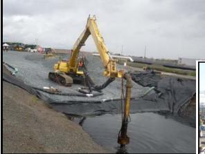
The Golden Eagle Refinery removed the oily sediments and backfilled the canal with clean rock and soil. The Refinery employed both mechanical excavation and hydraulic vacuum methods to remove the oily waste transport partially-treated refinery used to transport partially-treated refinery wastewater. After decades of operation, sediments in the canal were heavily contaminated.
