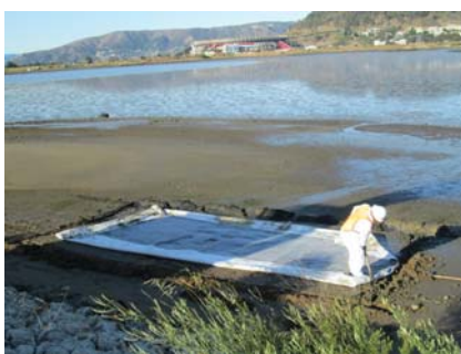
Photo 1b. July 24: Navy installs organoclay reactive mat over shoreline seep. Candlestick Park can be seen in the distance.
