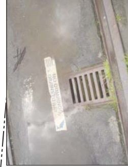
OPEN DRAIN TROUGH PIER SURFACE TO ESTUARY
