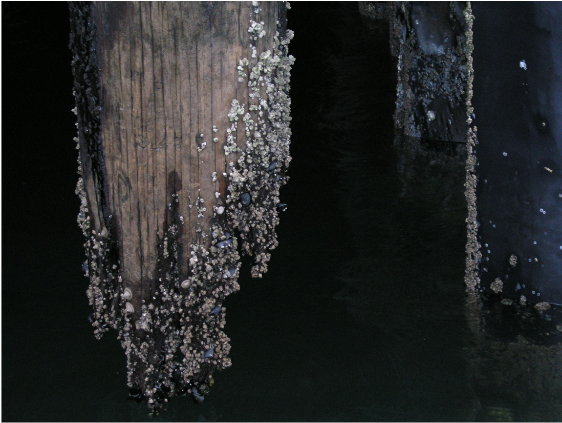
Figure 1. Broken pilings, hanging from the pier, were typical at the Ninth Avenue Wharf.
