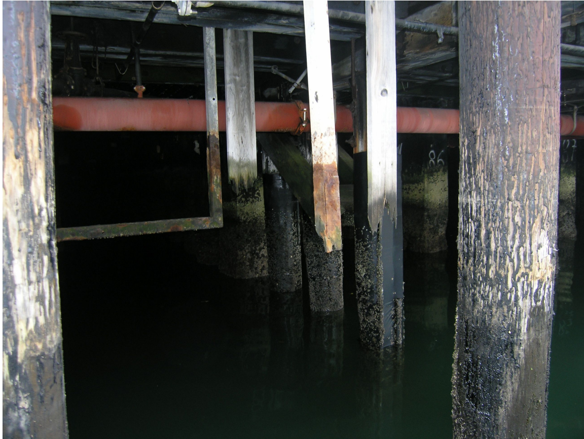
Figure 2. Many of the pilings at the Ninth Avenue Wharf are coated in creosote.
