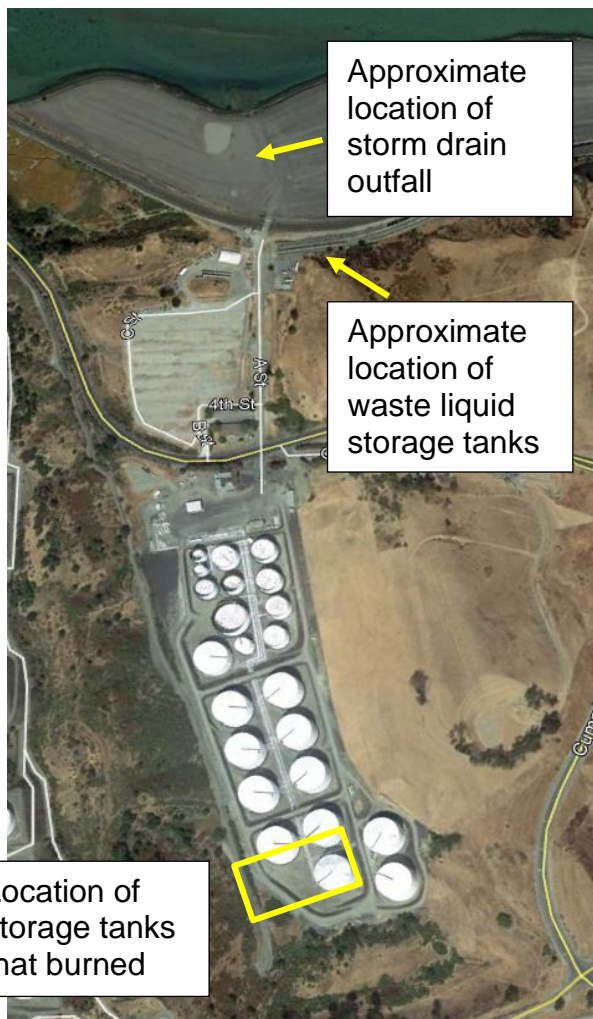
Figure 2: Location of aboveground storage tanks involved in fire and storm drain outfall at San Pablo Bay
