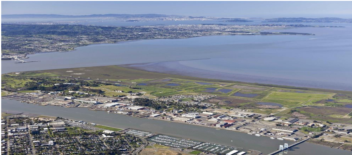
Aerial Photograph Showing Southern and Central Portions of Mare Island
