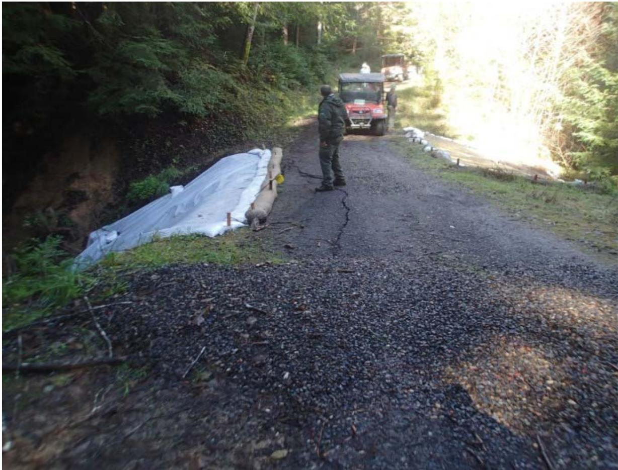
**Figure 3.** Cracking of Dark Gulch road prism around upstream sinkhole. The sinkhole has been covered with plastic tarp.
