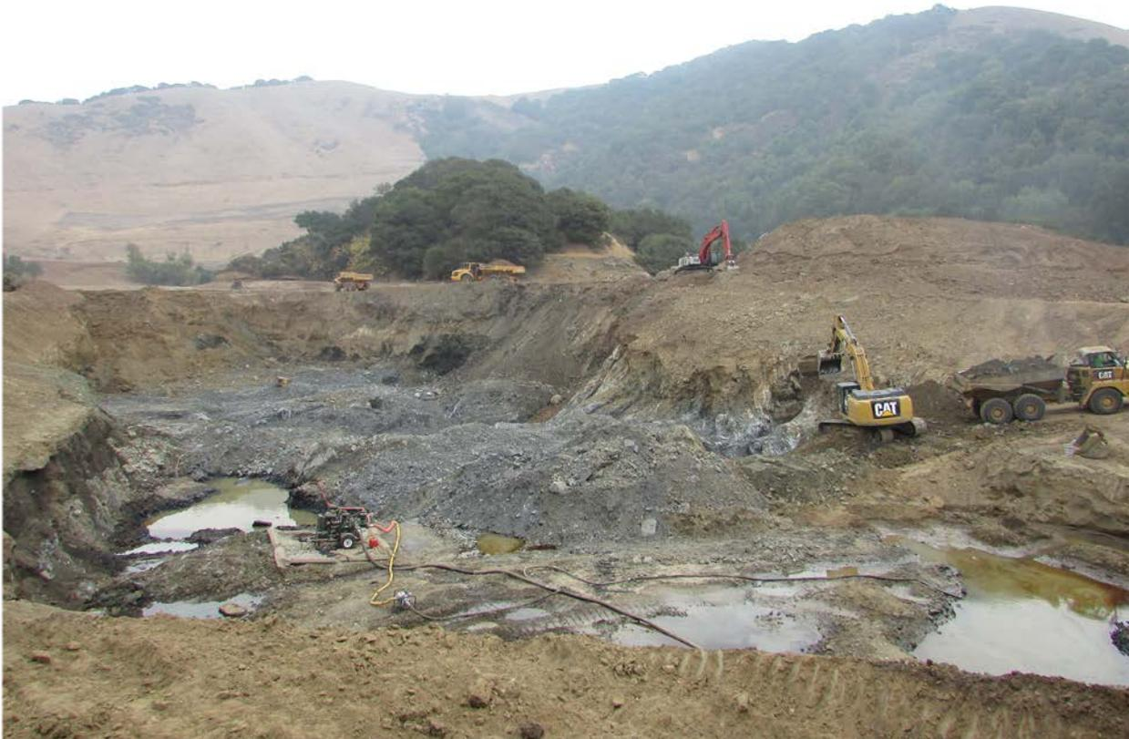
Figure 2 – Photo of onsite excavation. Note the bedrock surface.
