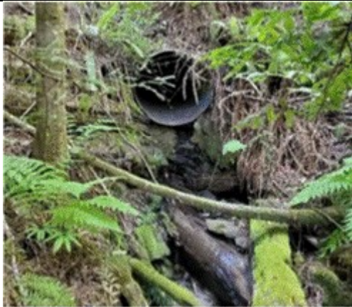
Figure 3: Old Haul Rd at Schenly Creek. Erosion undercutting the outlet of existing undersized culvert (48" diameter).
