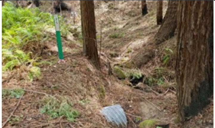
Figure 4: Old Haul Rd at Rhododendron Creek. Inlet of undersized 24" diameter culvert.
