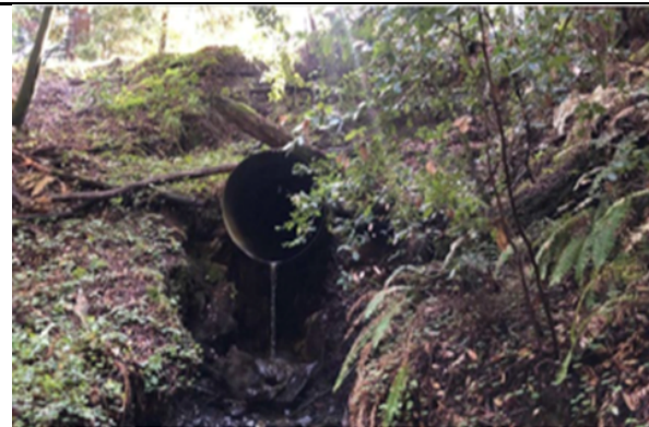
Figure 1: Wurr Rd. at Bloomquist Creek. Erosion undercutting the outlet of existing 78" diameter culvert.
