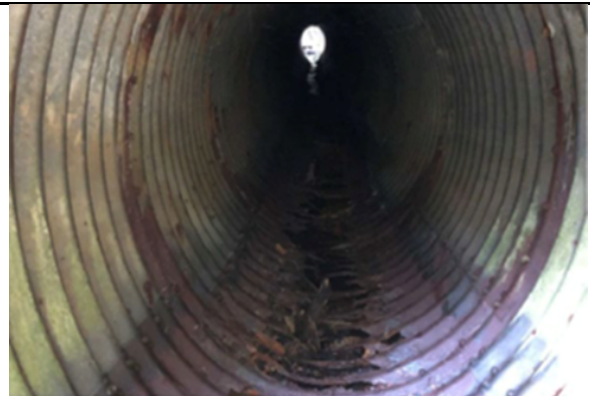
Figure 2: Wurr Rd. at Petersen Creek. Bottom of 84" diameter culvert shows signs of rusting out in 2021 and has continued to degrade.
