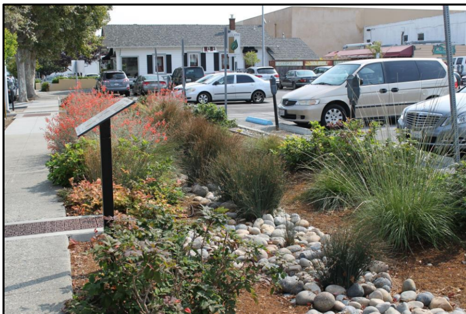
Figure 1: A bioretention system in the City of Burlingame designed to treat runoff from surrounding parking lots and other impervious surfaces. Bioretention systems function by allowing runoff collected from impervious surfaces during storms to pond to a specified depth and percolate through soil treatment layers before discharging to the MS4. This achieves pollutant removal via filtration and other removal processes, and reduces the rate that stormwater is discharged to receiving waters to reduce erosive flows and other physical impacts of hydrological cycle modifications due to urbanization. Source: C.3 Regulated Project Guide , Version 2.0, November 2023, San Mateo Countywide Water Pollution Prevention Program.
