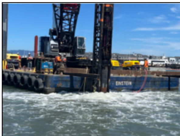
Figure 3: Sediment dredging at Pier 43 (Left); stability pile installation (Right).
