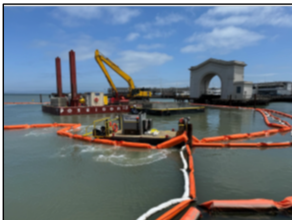
Figure 3: Sediment dredging at Pier 43 (Left); stability pile installation (Right).
