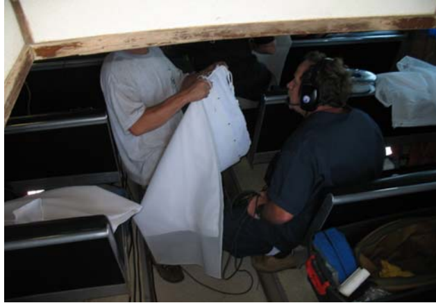
Figure 1 – Bags Being Secured Together
