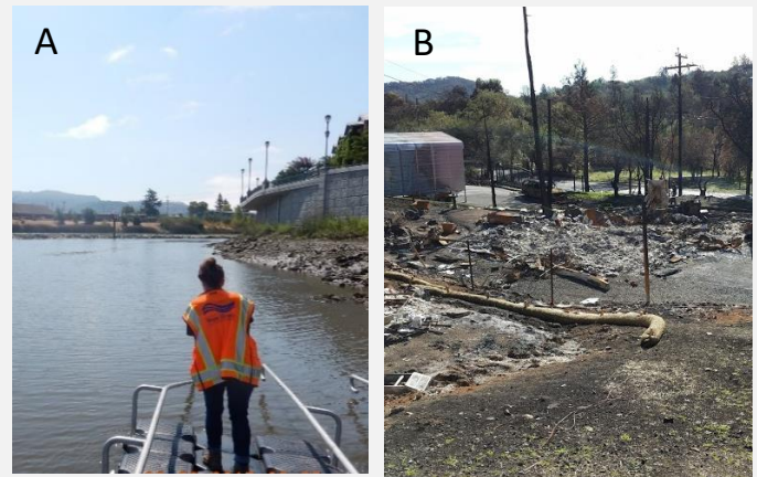
Figure 3. A) Water Board Staff collecting water quality samples at the Napa River in downtown Napa. B) Erosion and drainage controls installed next to a burned structure.
