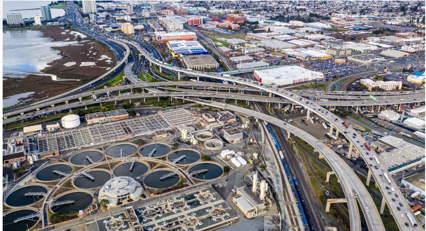
Conventional Plant at East Bay Municipal Utility District, photo SFEI 2025
