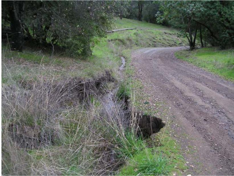
**Figure 4. Rills and Gullies on a Compacted Dirt Road**
