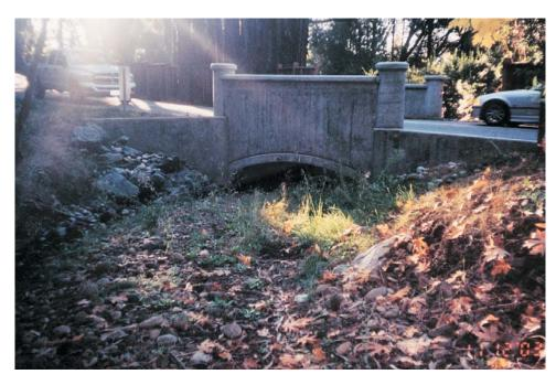
Site 11B Alambique Creek at 1990 Portola Road, looking downstream - note sediment accumulation blocking much of bridge opening
