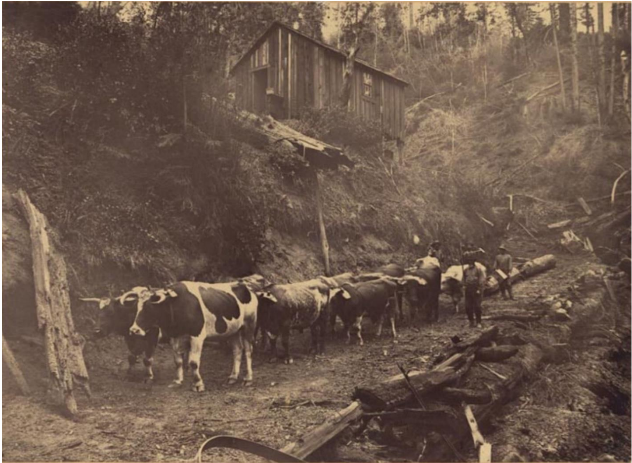
Figure 5.2 Oxen train hauling logs on corduroy road near La Honda (photo taken in 1881; Stanger 1967)
