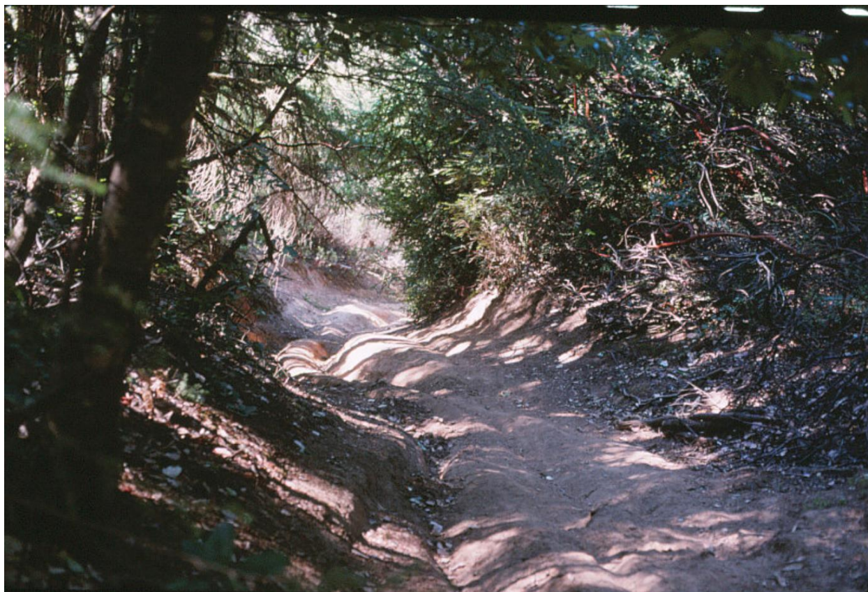
Figure 5.4 Abandoned throughcut logging road with deep rilling in the El Corte de Madera Creek Preserve (photo taken in 1994)
