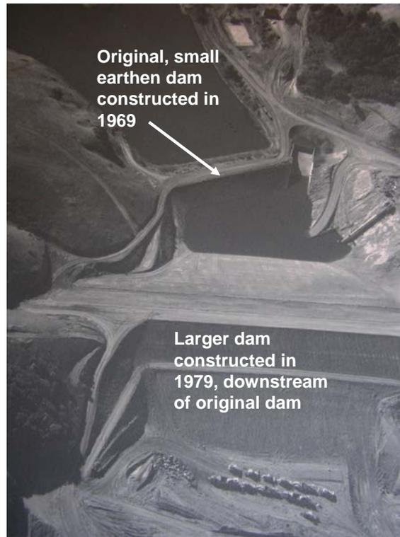
Figure 2. Original dam and construction of larger dam at Soulajule Reservoir. Source: MMWD.
