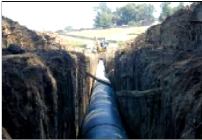
Figure 2-6: Drainage pipe installation at a vineyard in Mendocino County.
