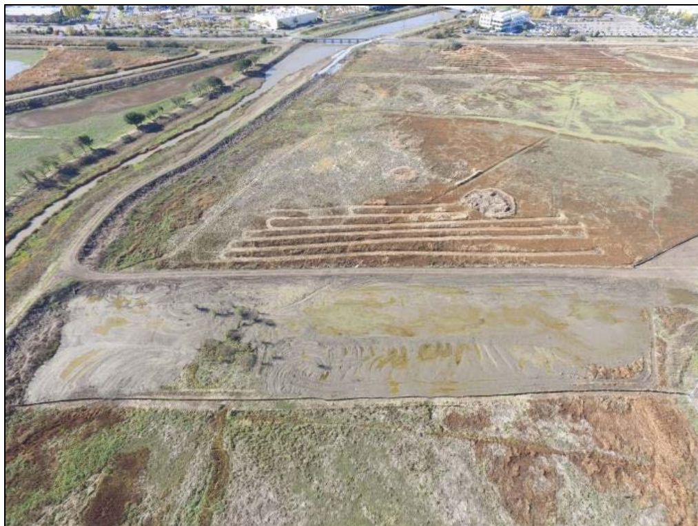
Figure 18. The new levee core and ecotone in Deer Island Basin shortly after construction in the fall of 2016. (Image: MCFCWCD)
