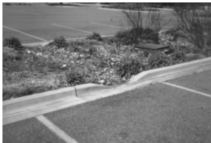
Figure 4. Bio-retention median or rain garden in Maryland with overflow drain visible on the right. The top of the overflow, shown here as a metal grate, is typically 9 inches above the bottom elevation of the bio-retention area.
