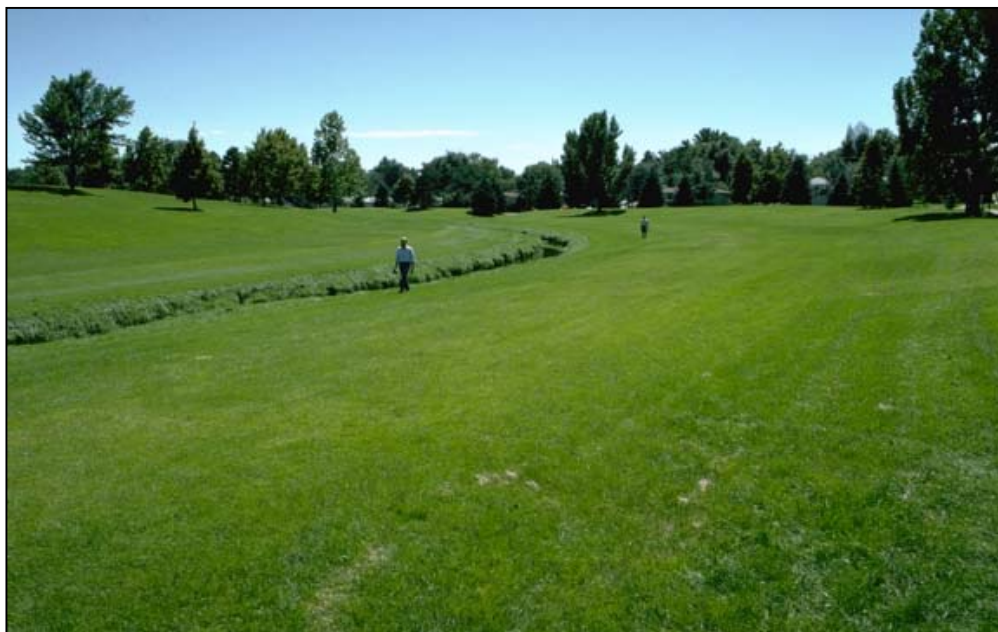
Photograph PL-5—A wide-open waterway carries floodwater at modest depths while maintaining low velocities to inhibit erosion.
