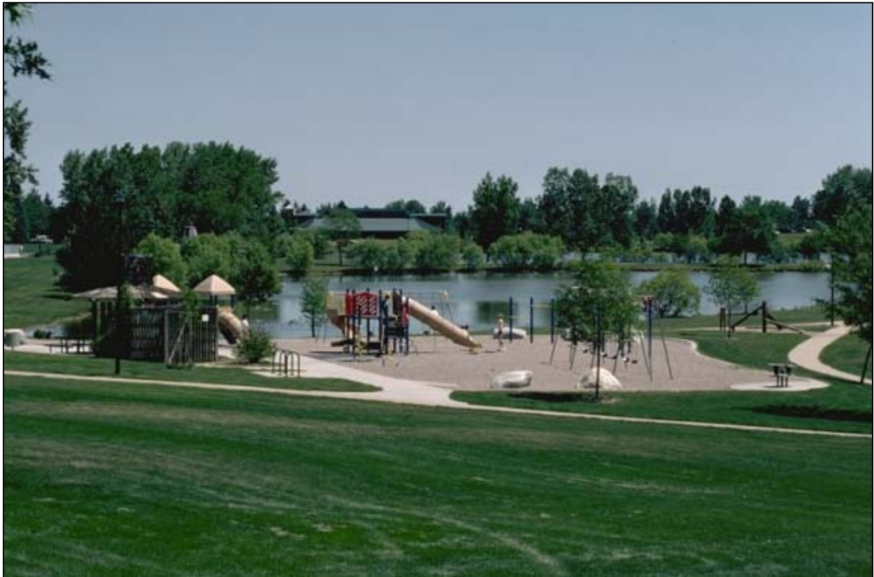
Photograph PL-7—Urban stormwater detention basins can create neighborhood amenities that at the same time serve their flood control function.
