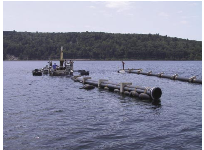
A barge helps position the pipe intake at the deepest part of the lake.
