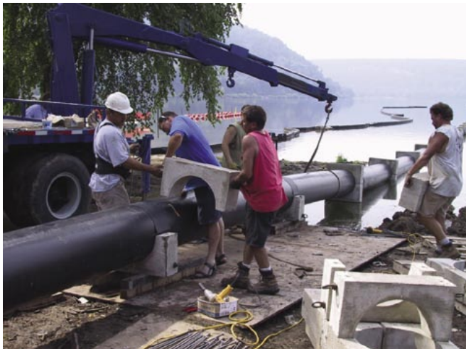
Concrete weights attached to the pipe keep it on the lake bottom.
