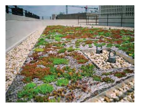
The first commercial high-elevation green roof in Washington, DC, will be monitored to determine how much it lowers air temperature.
