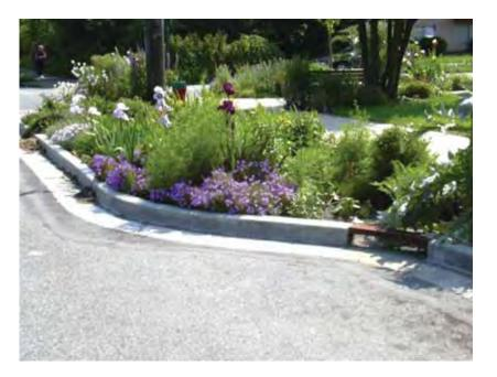
Infiltration bulges capture and infiltrate stormwater before it reaches the collection system. PHOTO COURTESY OF CITY OF VANCOUVER GREENWAYS PROGRAM
