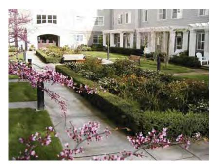
The vegetated infiltration basins in the Buckman Heights Apartments courtyard in Portland, OR, receive and infiltrate stormwater from building roofs and sidewalks.
