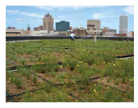
The green roof atop MMSD's headquarters, shown just after installation, demonstrates how stormwater flow into the city's sewer system could be reduced. PHOTO COURTESY OF MMSD
