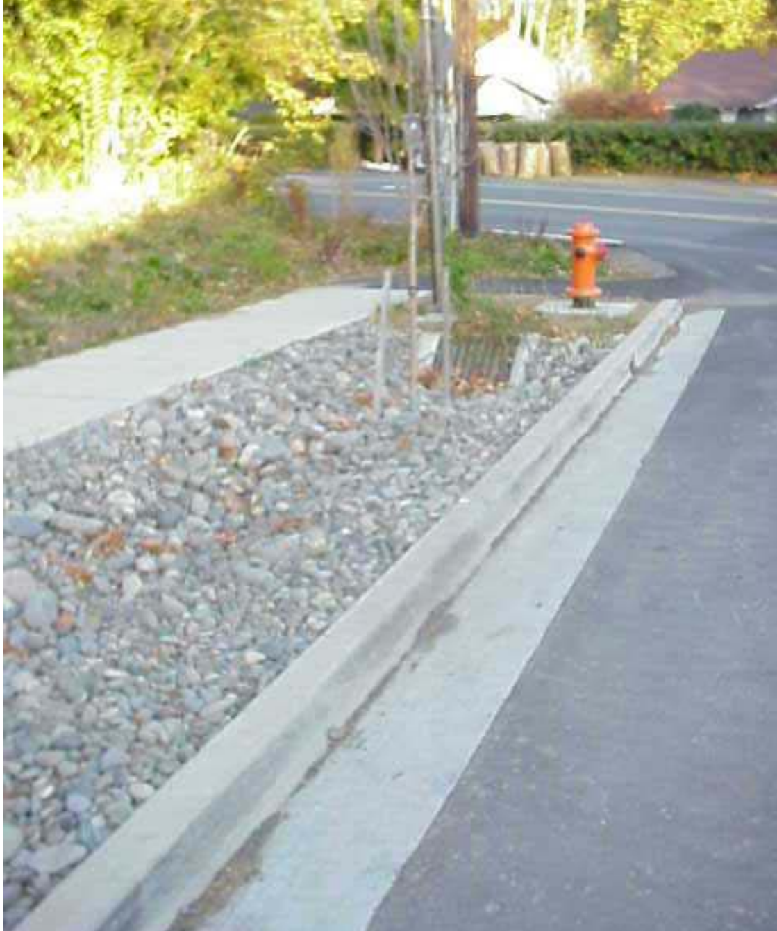
North side of SW Lodi Lane (& Shattuck), sand filter/ street swale
