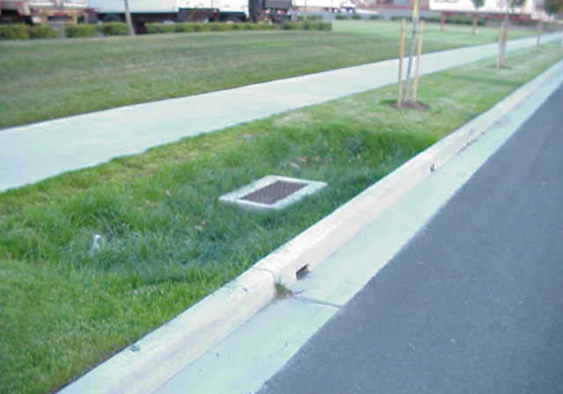
N Leadbetter Road street swale w/ overflow catch basin & curb slots
