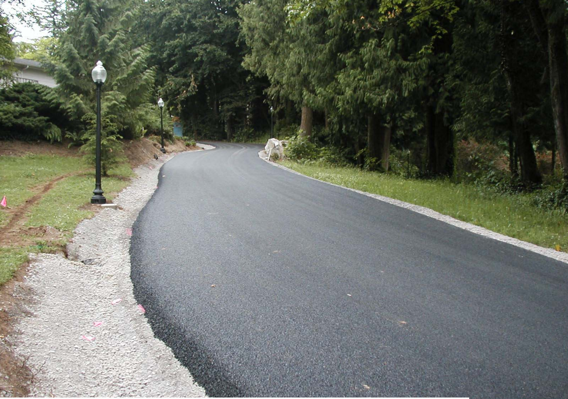
Pervious Asphalt installation near SE 162nd & Foster
