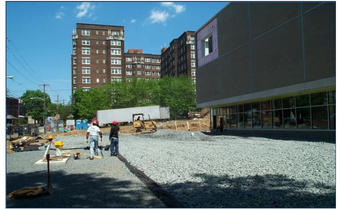
Figure 7: Penn Alexander School porous asphalt play yard under construction.
