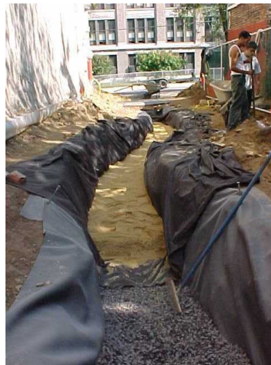
Figure 4: Construction of infiltration trench at Sulzburger Middle School demonstration site.
