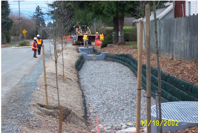
Figure 6. Construction of swale at 110 th Street cascade pilot project, Seattle, Fall 2003.
