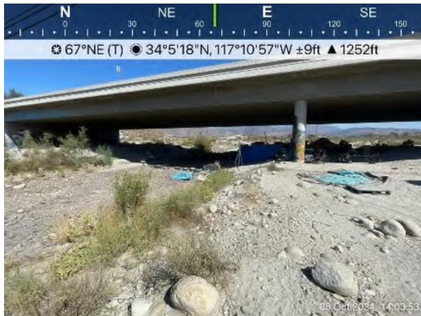
Figure 15: The upstream view from the middle of the "Drainage 4" reach.
