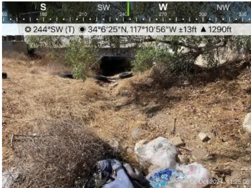
Figure 7: Downstream view from top of the reach of “Drainage 1A”.
