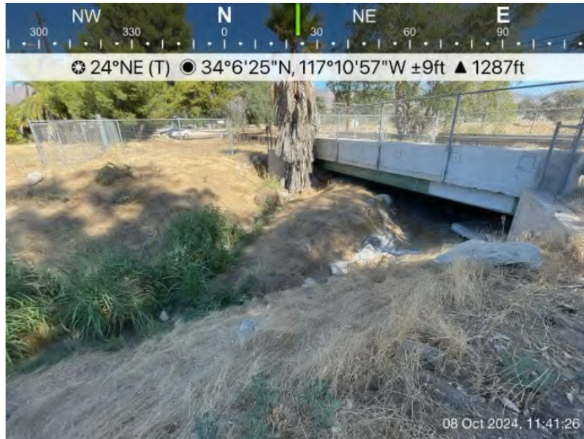
Figure 6: Overview of “Drainage 1A” and “Drainage 1B”.
