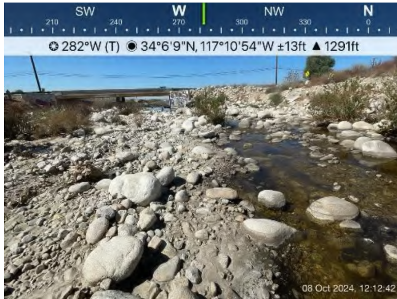
Figure 10: Downstream view from the top of the "Drainage 2" reach.
