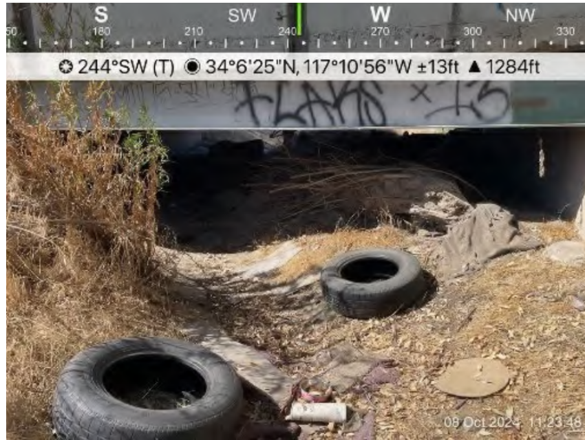
Figure 8: Downstream view from the middle of the "Drainage 1A" reach.
