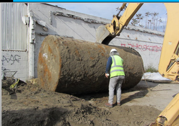
Photo 1: Removal of a gasoline UST
