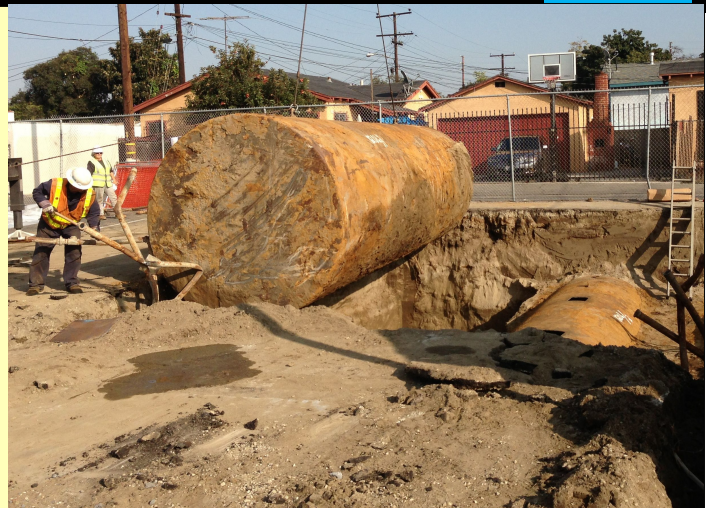
Photo 2: UST Removal in progress
