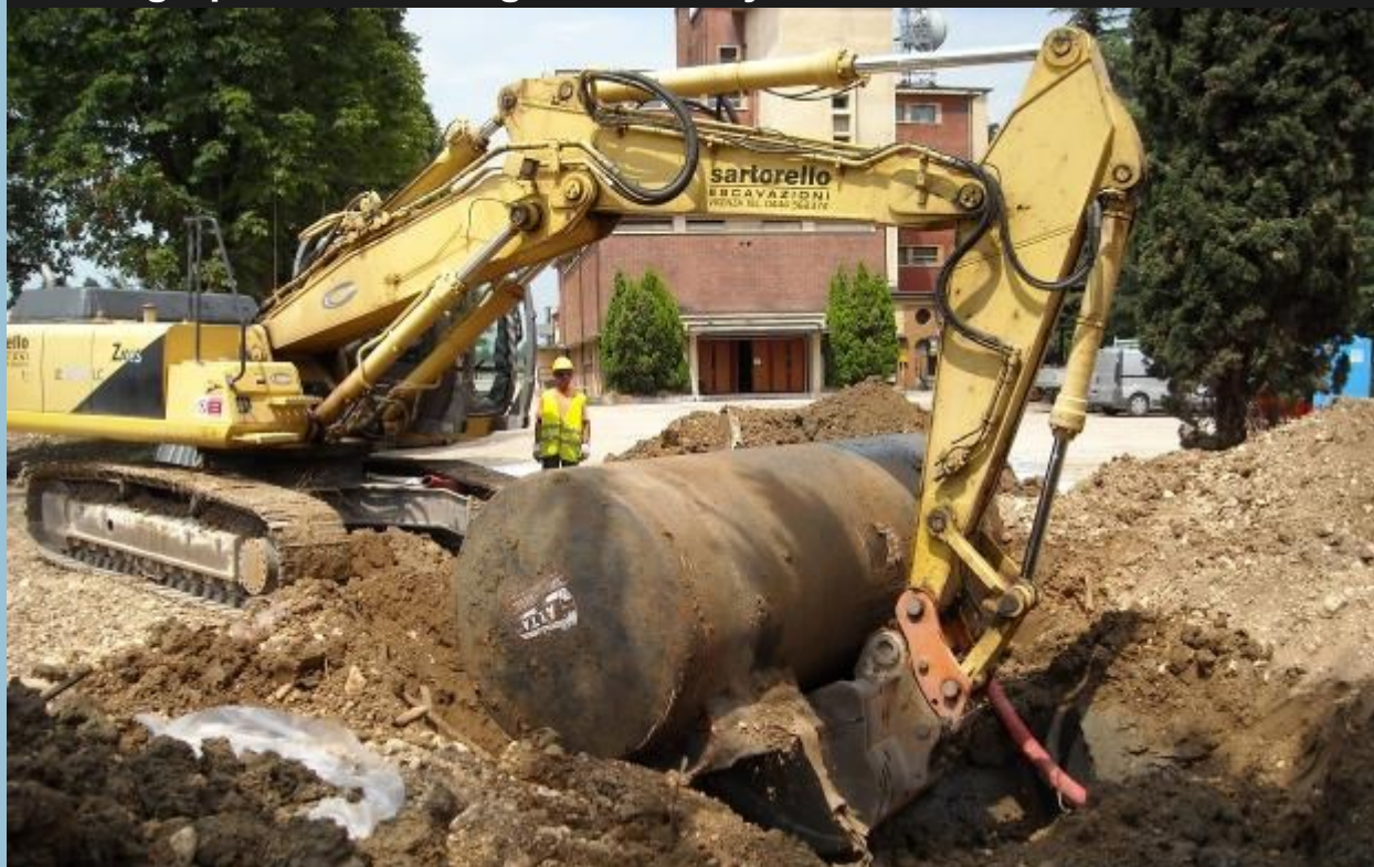
Photograph 1: UST being removed by a backhoe
