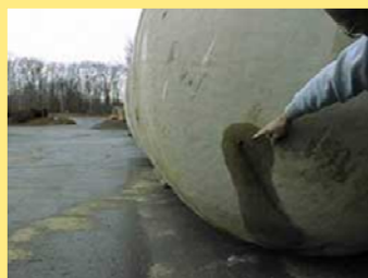
Removed formerly leaking and corroded UST.
