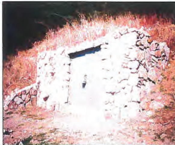
Figure 1-10. Bore Hole Enclosure at Spring No. 7
